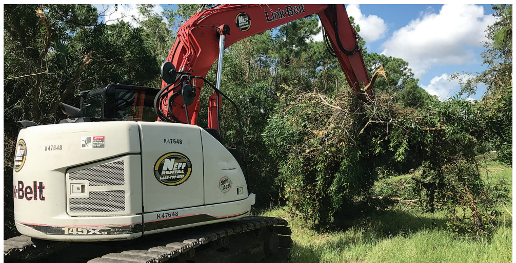
Hurricane Irma debris clearing
